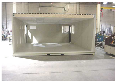
Two sections being test fitted at factory
