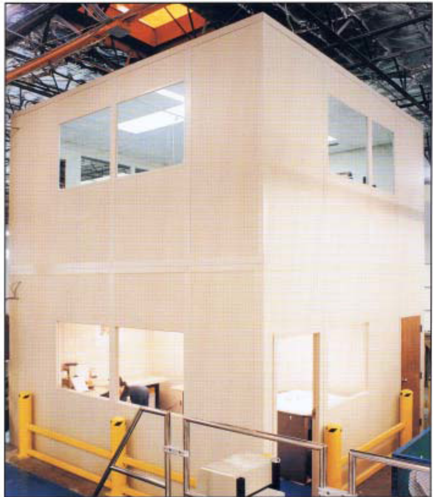
Clear Visions completed this pre-engineered two-story office (above) over a two-day weekend.
