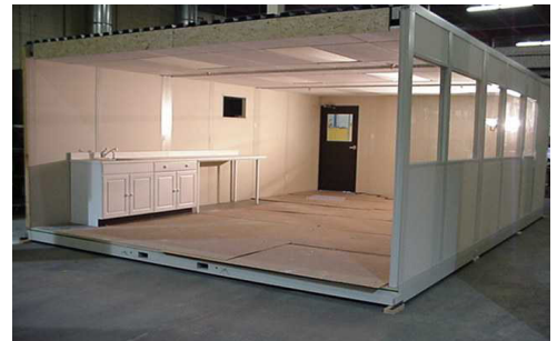
Room sections being test fitted at factory
