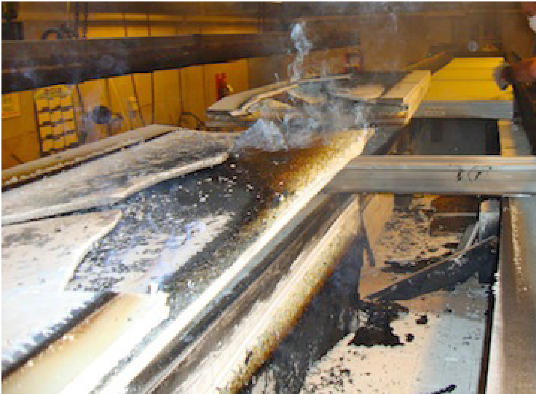
After 30-minute test: Showing exposed side of 1st 2 panels.
