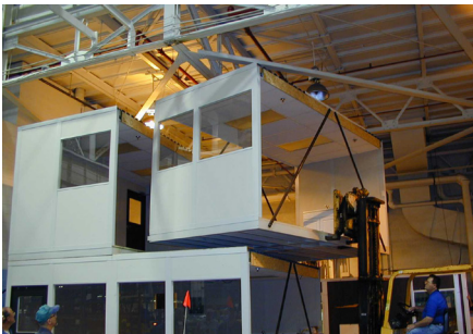
Room sections being set in place at jobsite
