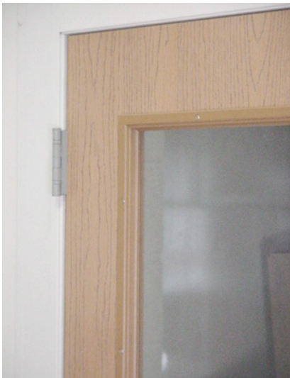
Finished Frame Front View Note that the frame is virtually invisible
